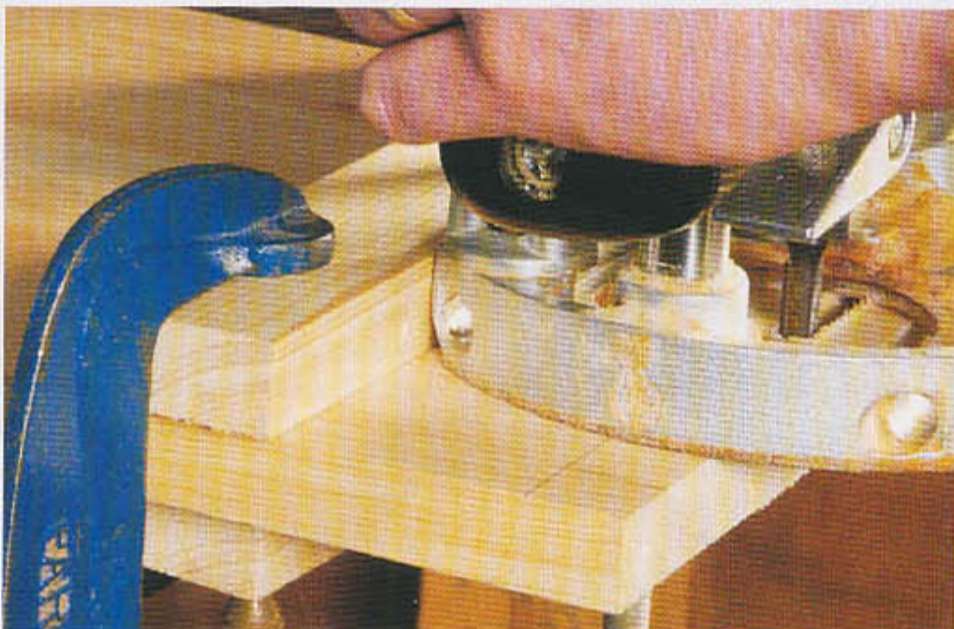
ABOVE & SECOND FROM BOTTOM - The trench and the tongue of the housing joint are cut using an electric router pushed against a wooden fence made from scrap wood
