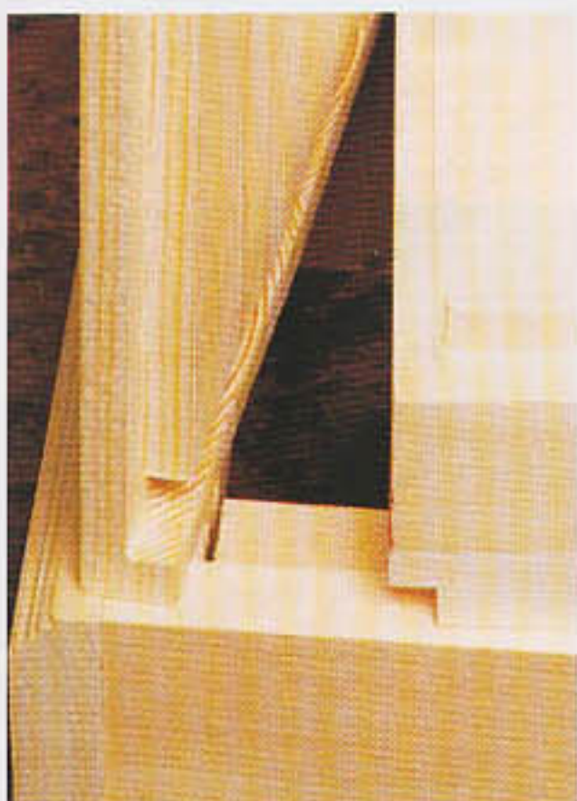
Detail of back showing the housing joint and rebate which holds the bead and butt boarding
