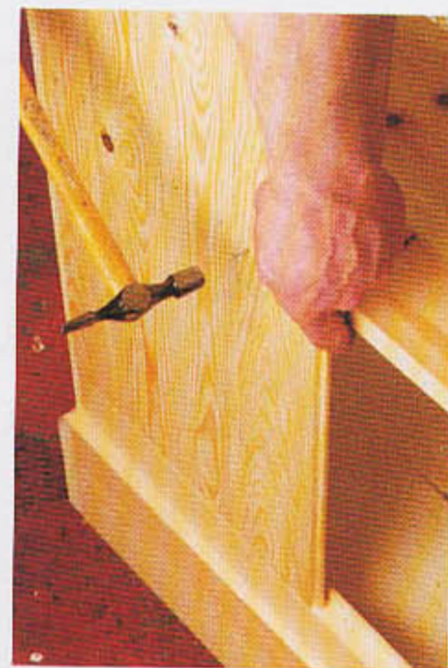
The bead and butt boarding is pinned into the back of the shelves
